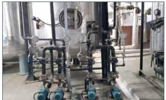
Circulation pumps with standby for hot water movement to swimming pool and rooms heat exchanger
