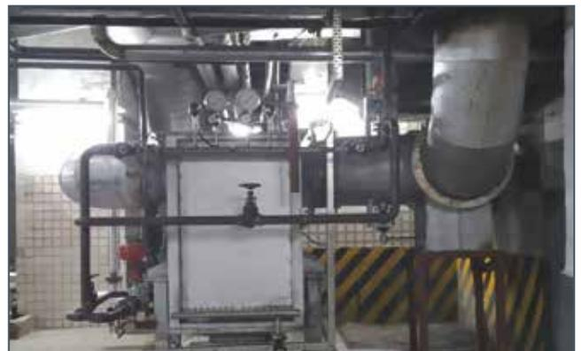
Water Pre-heater housing the ducting within its core
