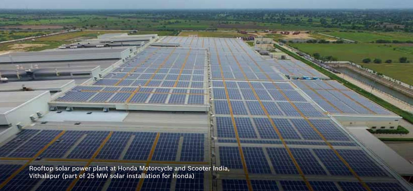
Rooftop solar power plant at Honda Motorcycle and Scooter India, Vithalapur (part of 25 MW solar installation for Honda)
