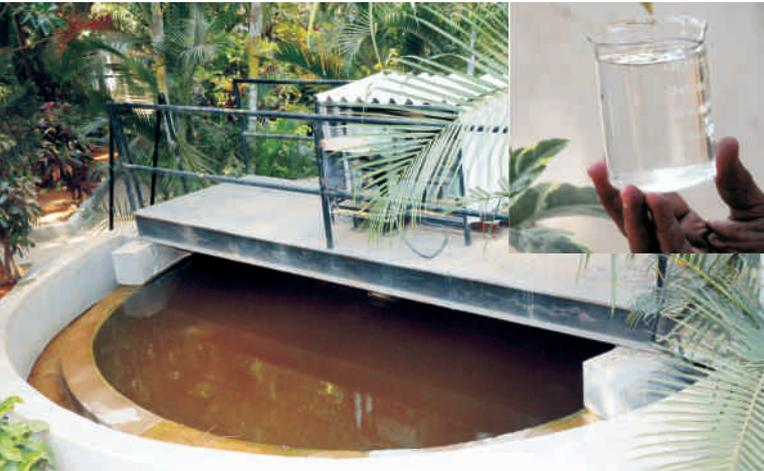
The clarifier at the canteen effluent treatment plant in Bangalore, which recycles and reuses domestic waste water.
