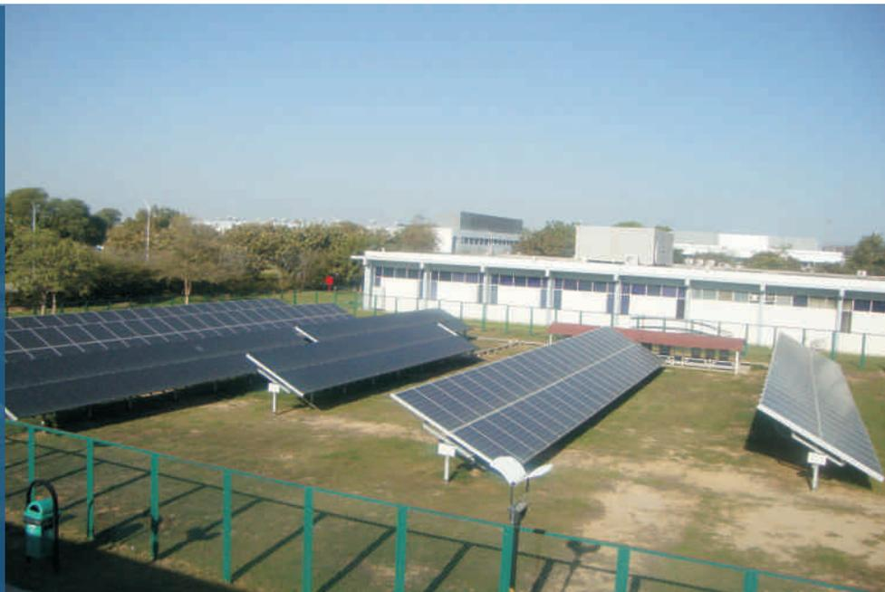
The Jaipur Plant's 40kW solar plant generates around 110 units of electricity a day.
