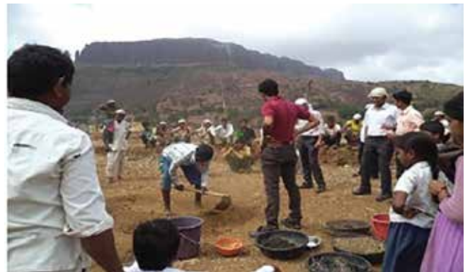
Figure 14: Villagers Working Hand-in-Hand with Bosch Team on Check Dam Project
