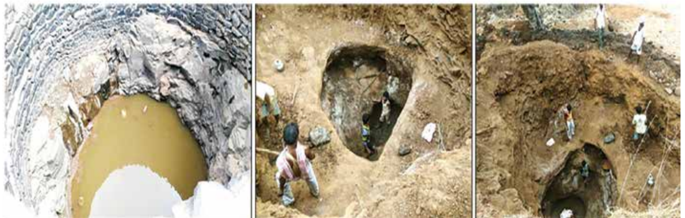
Figure 17: Storage Tanks: Before and After Situation
