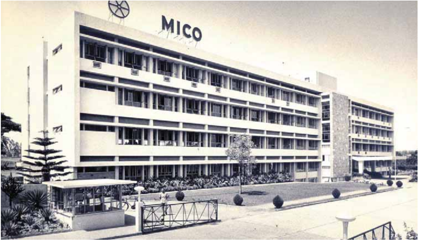
The newly-built administrative block of Mico (today Bosch Limited), Bangalore, in the year 1967.
